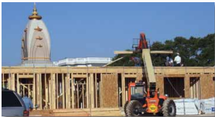
A team of workers erects framing for the new guest accommodations.
